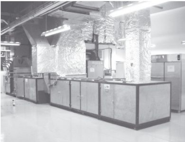
Figure 5.2 Cleanroom air conditioning plant
